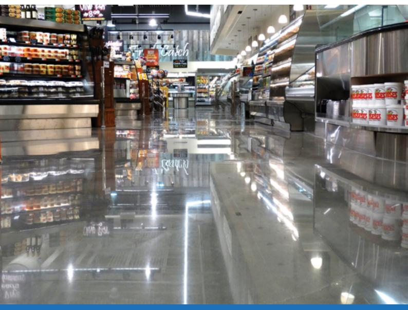
This reactive penetrating product forms an insoluble chemical bond to produce a dense sealed surface, with superior hardness, enhanced gloss and slip resistance.
