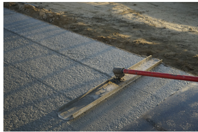
Apply first coat of SlabArmor Starter during float operations.
