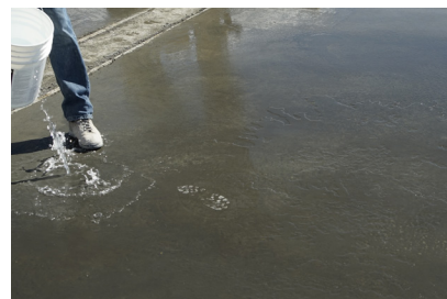
Unabsorbed material is washed off the slab.
