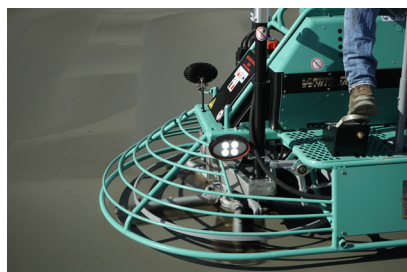
Trowel concrete to desired surface texture.
