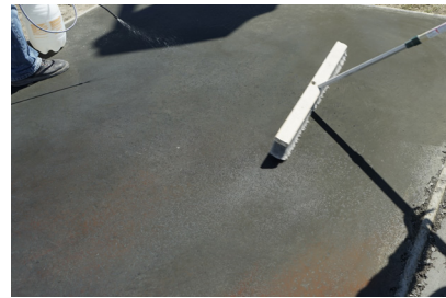
After the concrete floor has sufficiently hardened, Sodium Silicate is applied.
